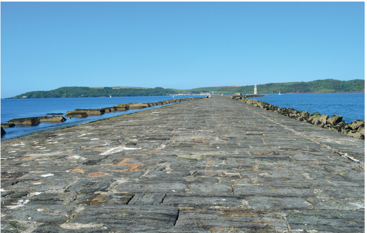
Above and Below: The Breakwater is surprisingly wide, its edges gently sloped to minimize damaging impact by the sea, whilst extracting the energy out of the waves. An additional line of huge blocks were later added along the south-facing seaward edge, dropped in place using specially designed cradles to lift and drop such heavy stones.
