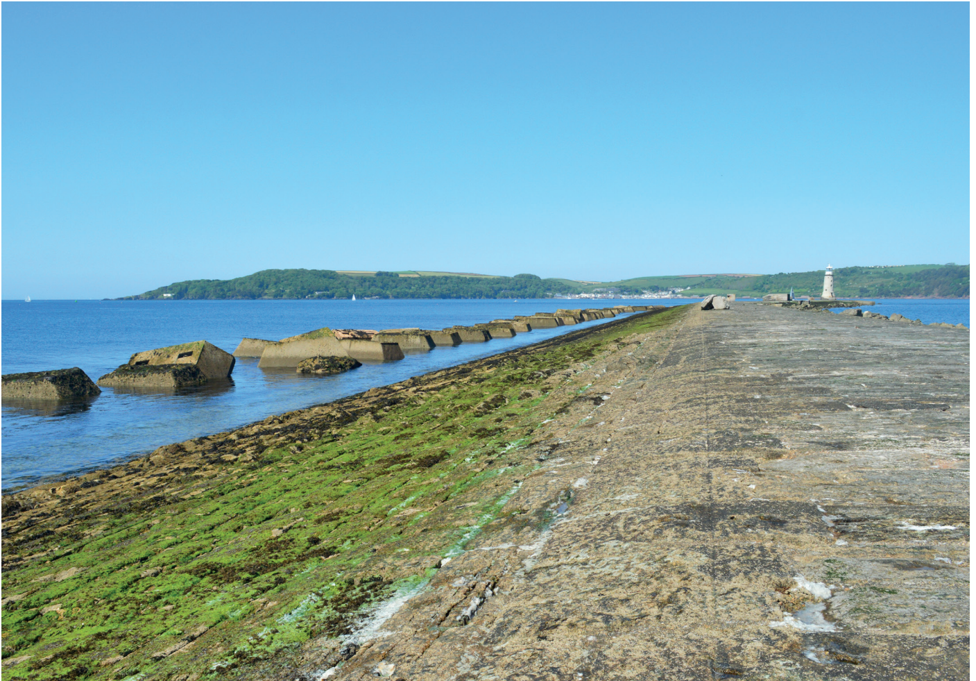
Above and Below: The Breakwater is surprisingly wide, its edges gently sloped to minimize damaging impact by the sea, whilst extracting the energy out of the waves. An additional line of huge blocks were later added along the south-facing seaward edge, dropped in place using specially designed cradles to lift and drop such heavy stones.
