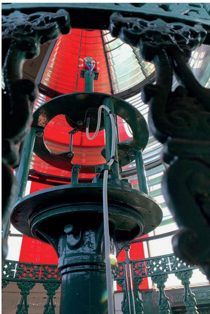
Above: The original pedestal remains in place inside the optic. A cable provides the electricity for the lamp. Below: The landward side of the optic has a cut-out section to give access to the light source. We note that the flue that would have carried away the gases - products of combustion of earlier paraffin lights - is also still present, leading up to its joint with the roof.
