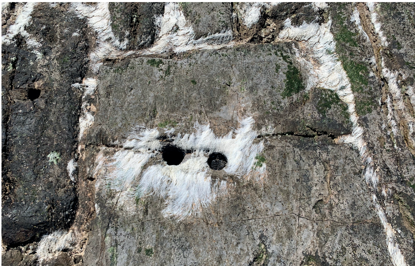
Below: Many of the stones have holes used to facilitate placement. White whiskers of a marine growth are everywhere.
