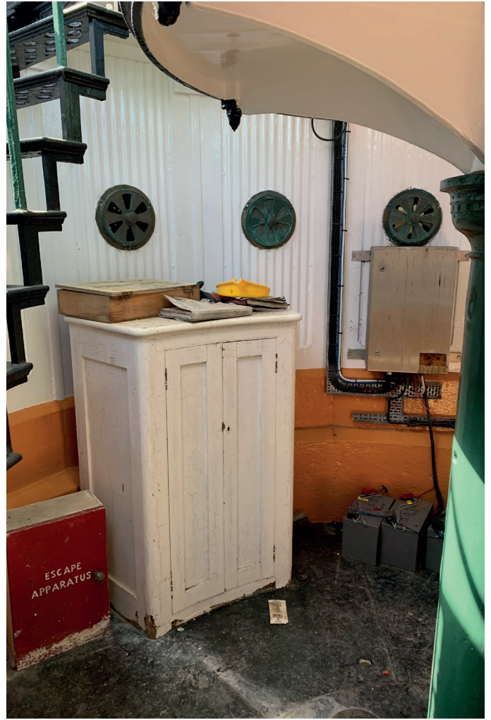
Above: The lower lantern area contains batteries to supply the light in emergency. Air vents around the inside wall are seen around the white-painted cast-iron lower part of the lantern.
