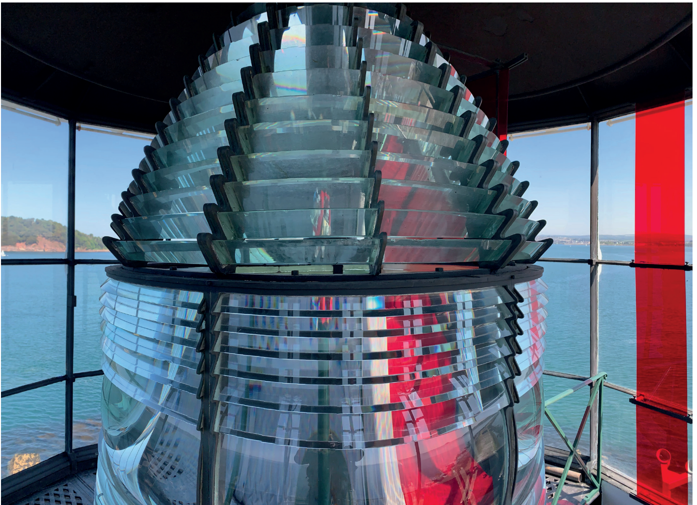
Above: The optic - known as a 'beehive' - is complete from this angle, but has a cut-out section on the reverse side that enables access for maintenance and visitors like me to look at the light inside.
