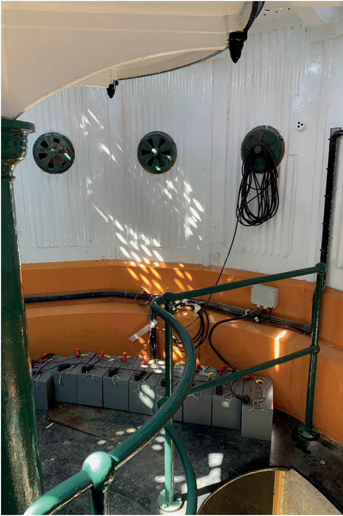
Above: The lower lantern area contains batteries to supply the light in emergency. Air vents around the inside wall are seen around the white-painted cast-iron lower part of the lantern.
