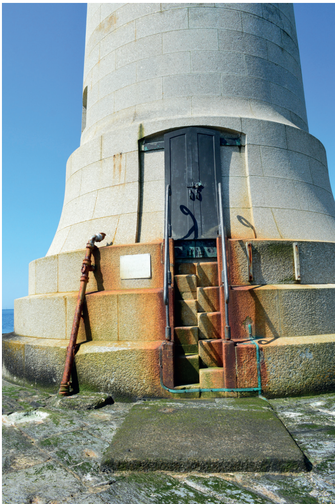
Below: The entrance as it is in 2023. The two gunmetal doors are very heavy and slide in horizontal tracks.
