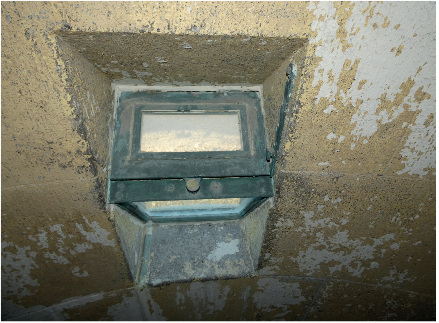
Above: The smaller windows of the service room are of two angled panes set in gunmetal. [Photo: Ruth Drinkwater.] Below: The stairs leading down from the service room to the bedroom. [Photo: Ruth Drinkwater.]
