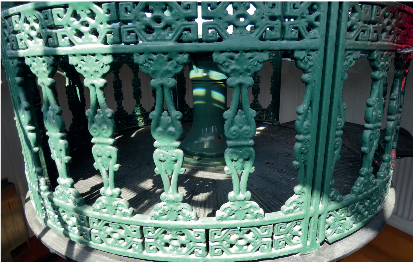
Below: The magnificent cast-iron pedestal on which the beautiful optic is mounted. [Photo: Ruth Drinkwater.]
