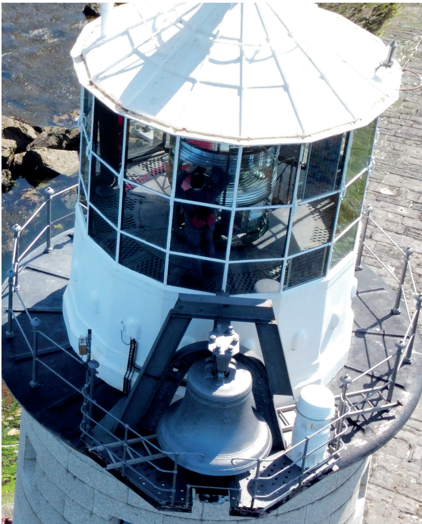
Above: This photo perfectly shows the old fog bell that was in use until 1994, when it was replaced by the modern white unit on the balcony in the lower right corner of the photo. [Photo: Nick Tadd]
