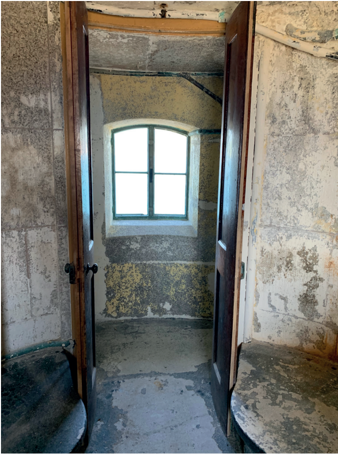
Level 2: This was originally called the oil store - two half-doors at the entrance because there is no room for a single door. The purpose of the unique, kidney-shaped plinths is curious, apart from elevating containers that need to be raised off the floor, as is the case with what looks like a water tank on the right, below.
