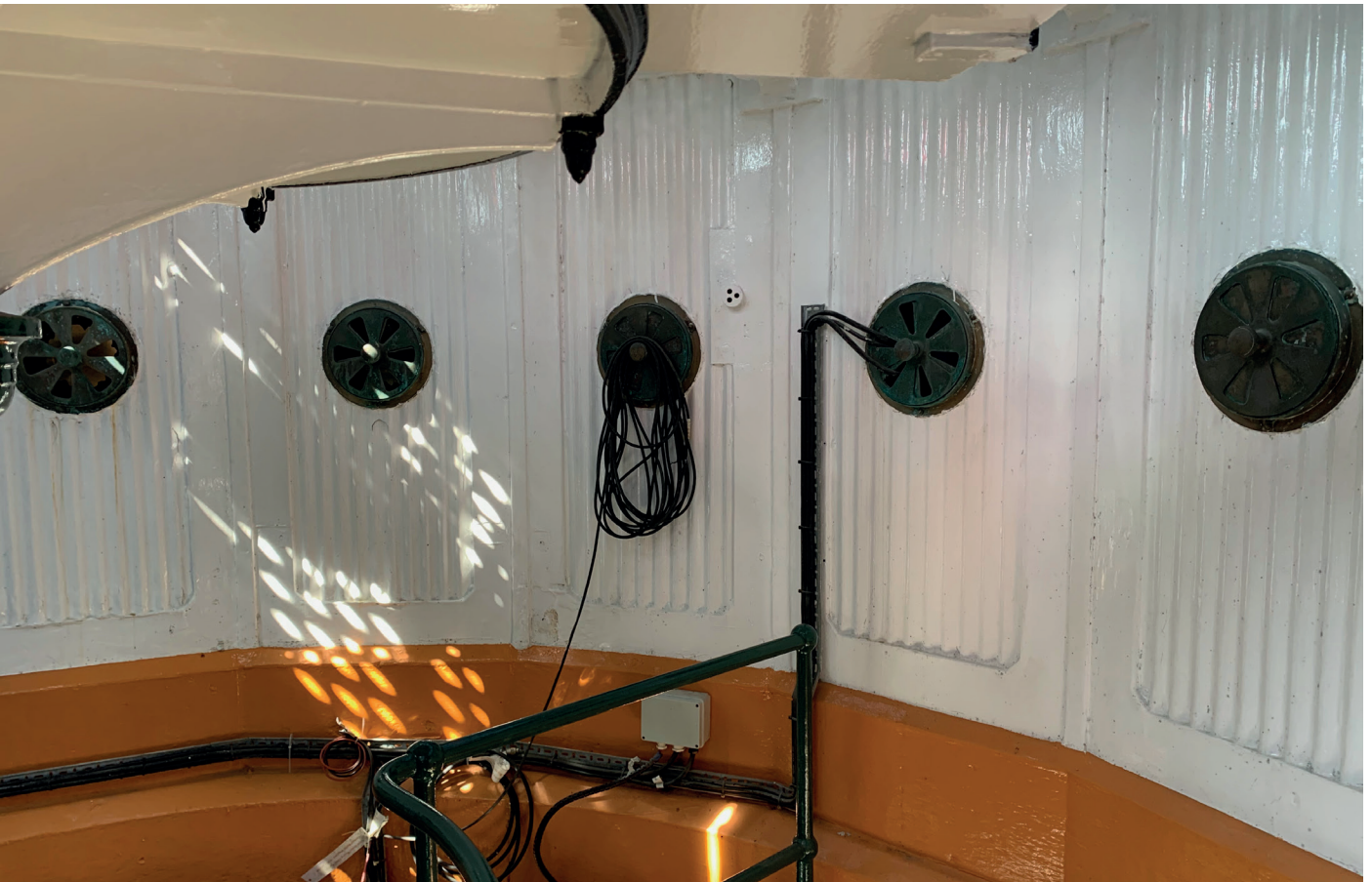
Above: The steps leading down from the lantern room to the service room. The pedestal of the optic is on the left. Below: Ventilators in the wall of the cast iron lantern.
