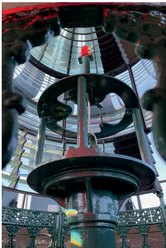
Above: The original pedestal remains in place inside the optic. A cable provides the electricity for the lamp. Below: The landward side of the optic has a cut-out section to give access to the light source. We note that the flue that would have carried away the gases - products of combustion of earlier paraffin lights - is also still present, leading up to its joint with the roof.
