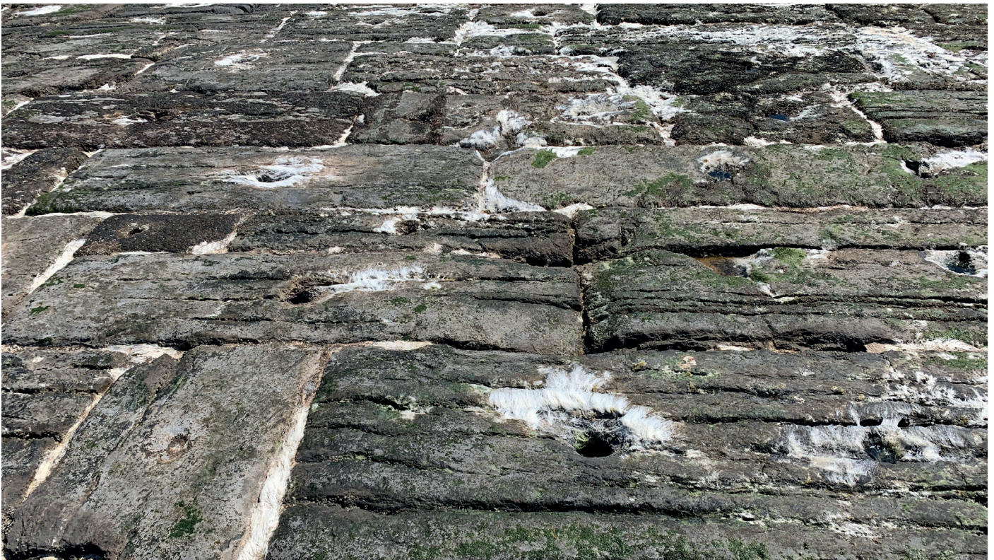
Above: The central part of the Breakwater has extra reinforcement that once formed a harbour for supply of stone. Below: A typical view of the top surface of the Breakwater shows the interlocking stones.
