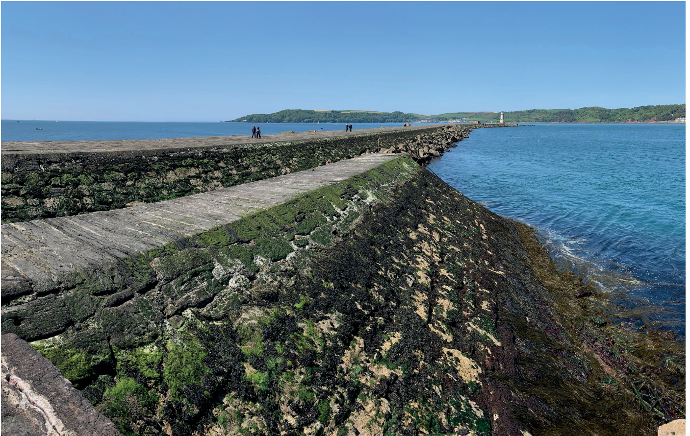
Above: The central part of the Breakwater has extra reinforcement that once formed a harbour for supply of stone. Below: A typical view of the top surface of the Breakwater shows the interlocking stones.
