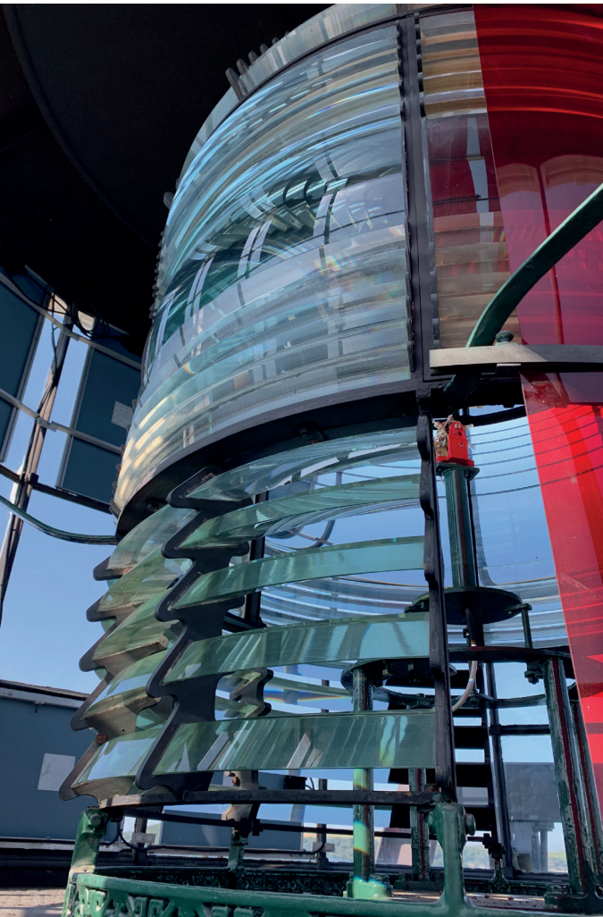
Views of the original optical apparatus. Unlike the situation in some other lighthouses, there are no rotating parts of the light mechanism. The optic remains in a fixed position and the light is switched on and off by electronic control.
