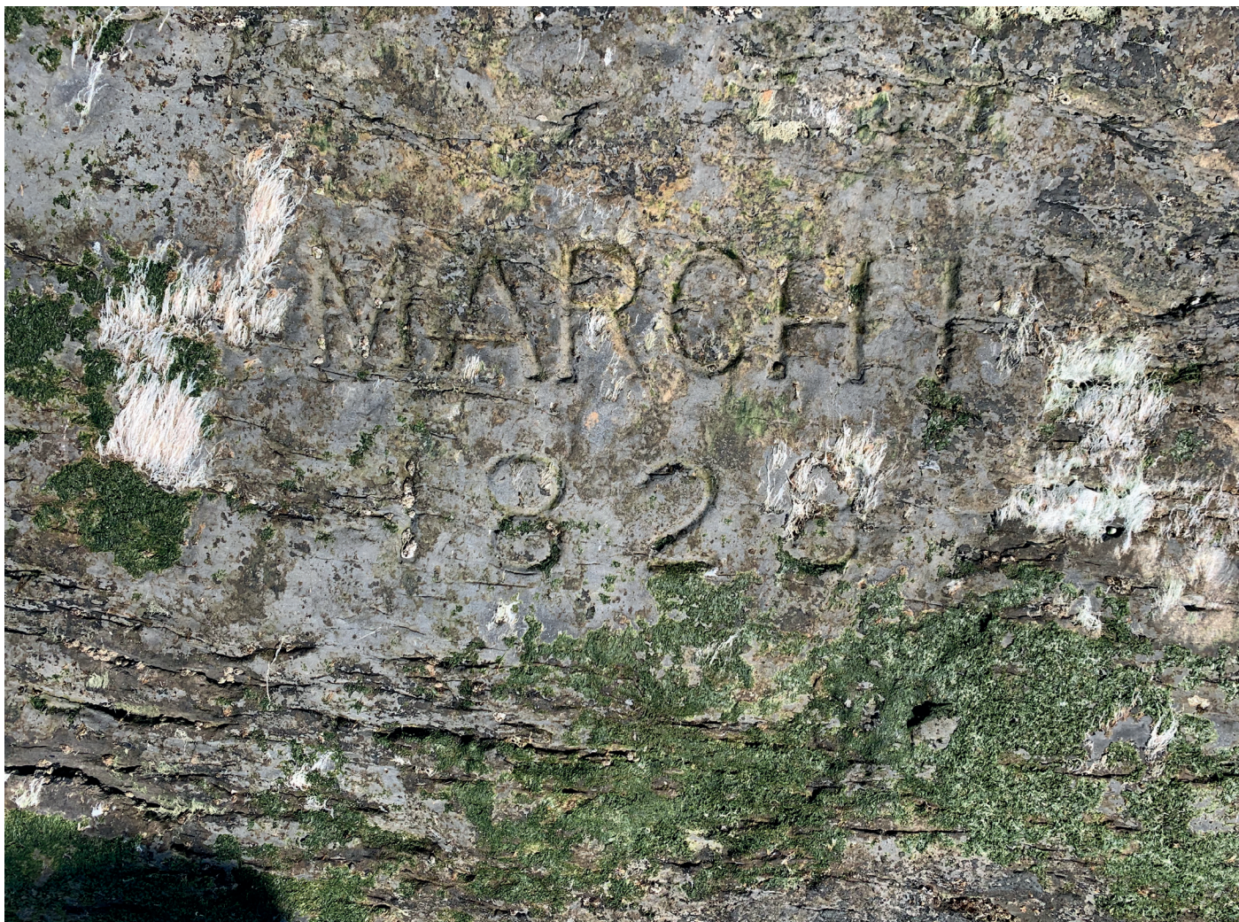
Above: One stone has March 1828 engraved into it, laid during the course of the build.
